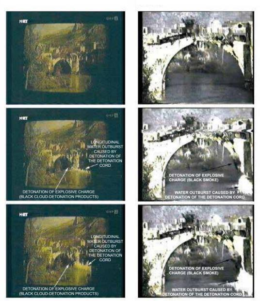
Picture 7. Chronological sequence of the occurrence of the water gush and the explosion at the bottom of the bridge arch.
